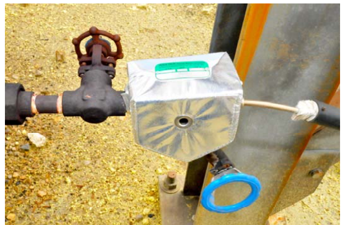
( 20 DN ) Gestra®Model-MK45 Thermostatic Steam Trap
