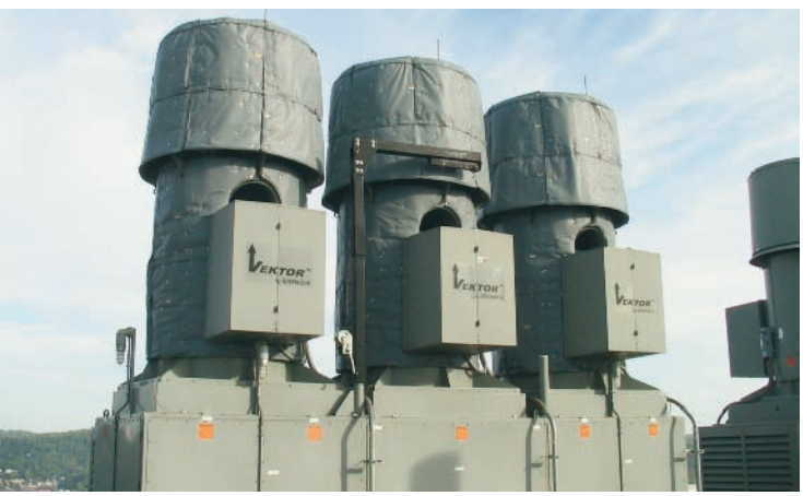
AXIAL FAN HOUSING Design: LT450A-TT - 1.5" thick - Wiretwist / Velcro® Flap Fasteners 6 dBA Reduction
