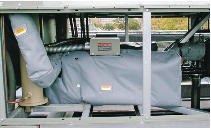
SCREW COMPRESSOR & DISCHARGE PIPING Design: LT450A-TT - 1.5" thick 6 - 8 dBA Reduction
